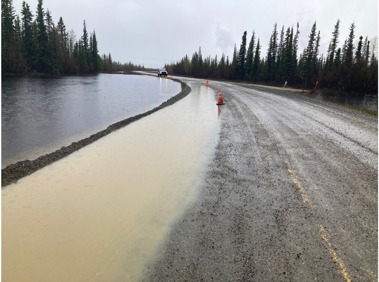
Picture of flooding on Northway Rd.
